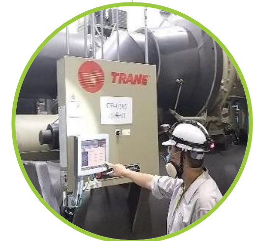
Chiller equipment maintenance
