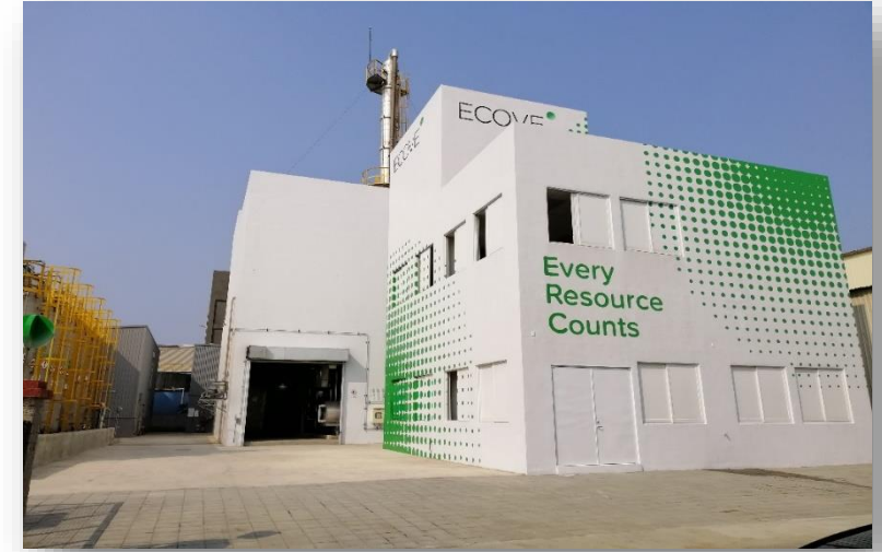
ECOVE SRC Waste Isopropanol Recycling Plant
