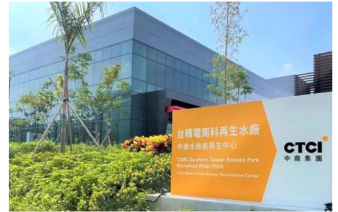
TSMC Southern Taiwan Science Park Reclaimed Water Plant
