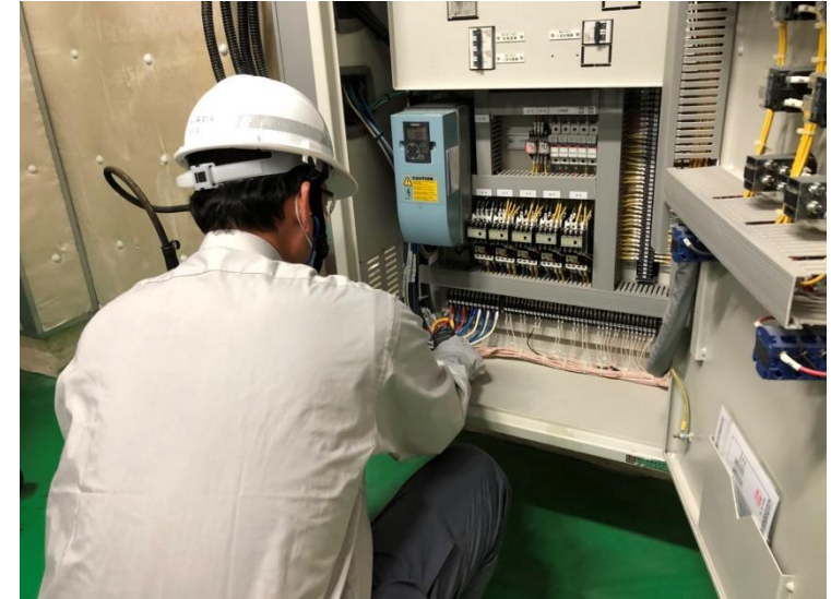
Air conditioning equipment maintenance
